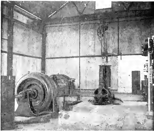
FIG. 5.—FIRST GENERATOR INSTALLED.
